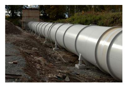
Figure 4. Straight penstock down-stream surge chamber
